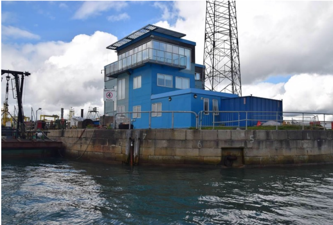
Plate 3-6 Pier Head at the terminus of Breakwater Road and the Port's Operations Building
